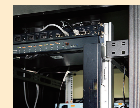
5. Z bracket, mounting style 2
