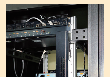
5. Z bracket, mounting style 2
