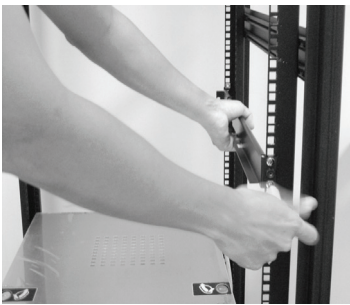
1. Secure the side rails to the rack.
