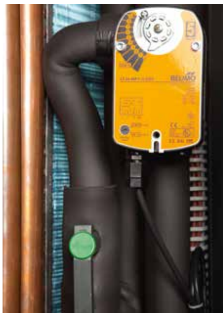
Switchover between a 2 and 3-way valve
