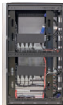
Side view of HP rack with modular PDU mounted in OU (on side)
